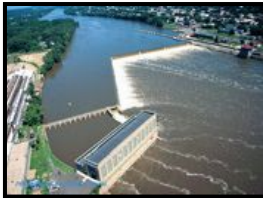
Green Island Hydroelectric Power Plant
