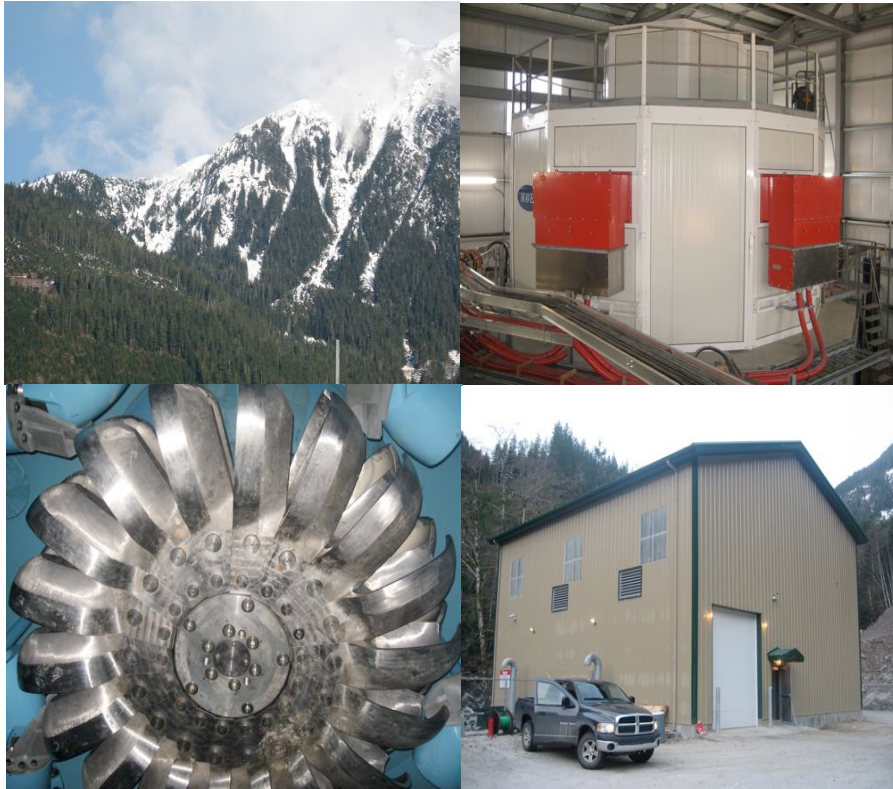
Clockwise from top left: Site, Inside Powerhouse, Mavel Pelton runner, Powerhouse
