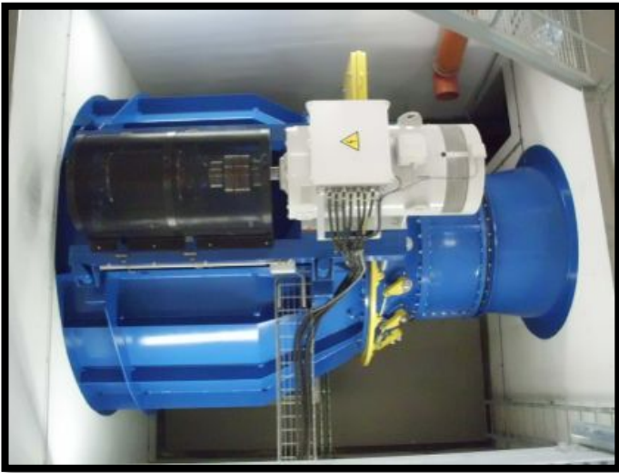
Kaplan Turbine in the Machine Room
