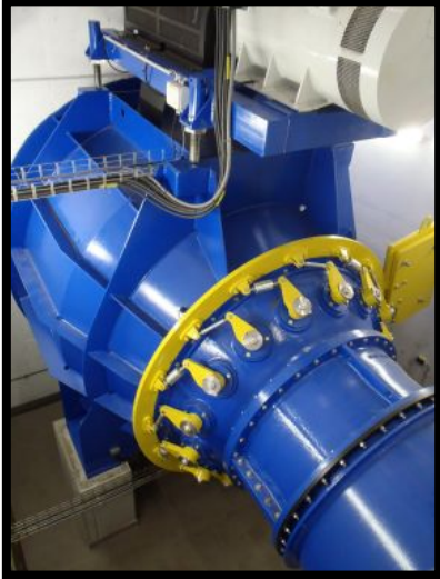
Installation of the Kaplan Turbine
