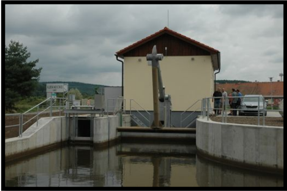
The Hluboka HPP Powerhouse
