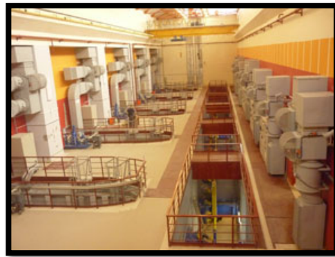
Interior of the Powerhouse
