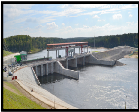
Completed Grodnenskaya HPP
