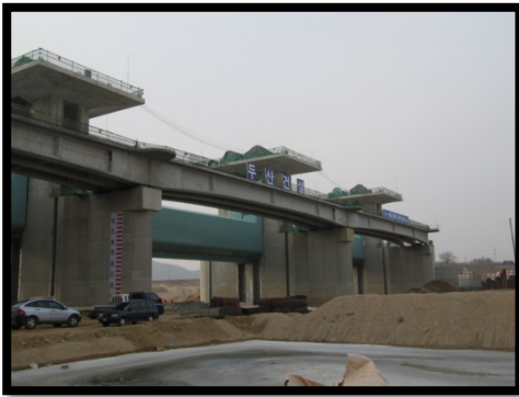
The Nakdan HPP under construction
