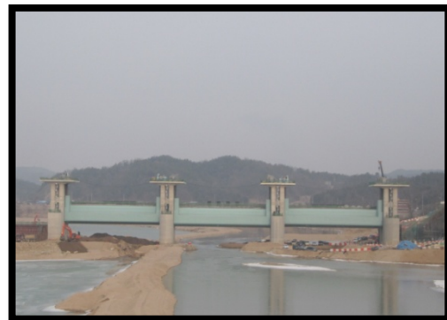
The completed Nakdan HPP
