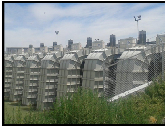
Eight Mavel TM10 Turbines Installed at North Side Canal Co.'s Head of the U Irrigation Project
