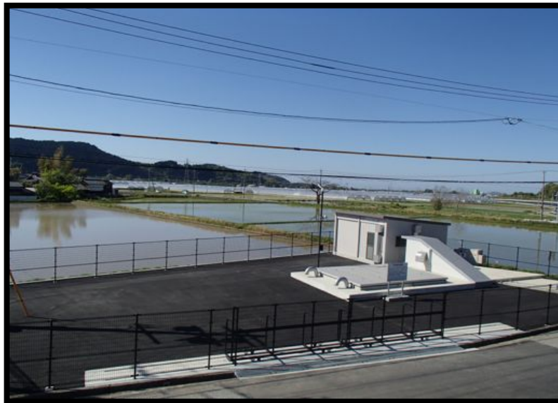
The view onto irrigated rice fields over the Yamada HPP Powerhouse
