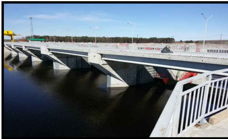
The Weir at the Polotskaya HPP
