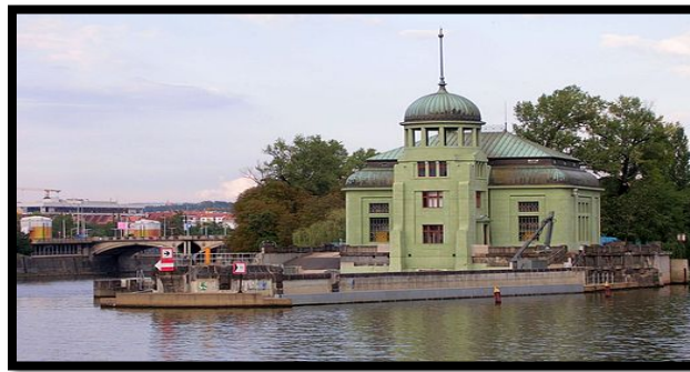
Prague’s Štvanice Hydroelectric Power Plant
