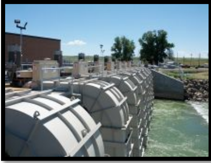
Head of the U HPP, USA 8 x TM10 Turbines
