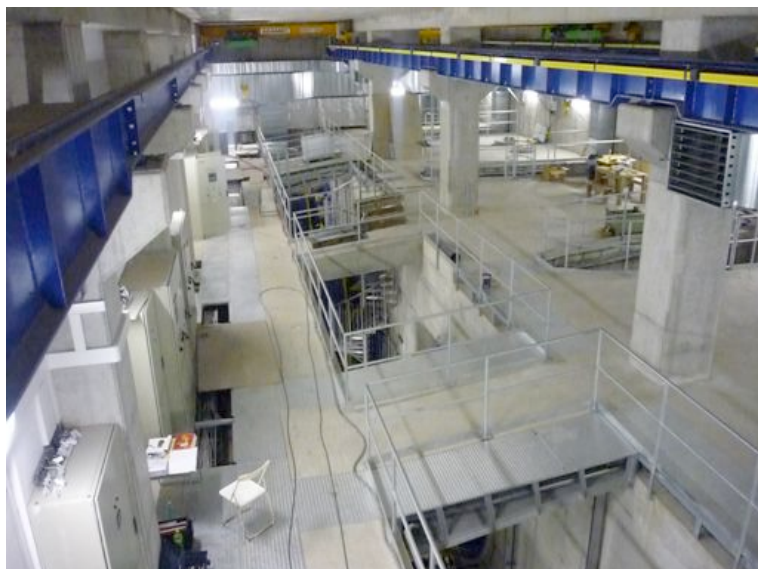
The interior of the new Lovosice HPP powerhouse
