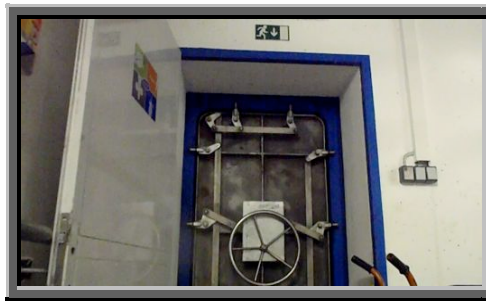
Access door at Lovcise HPP
